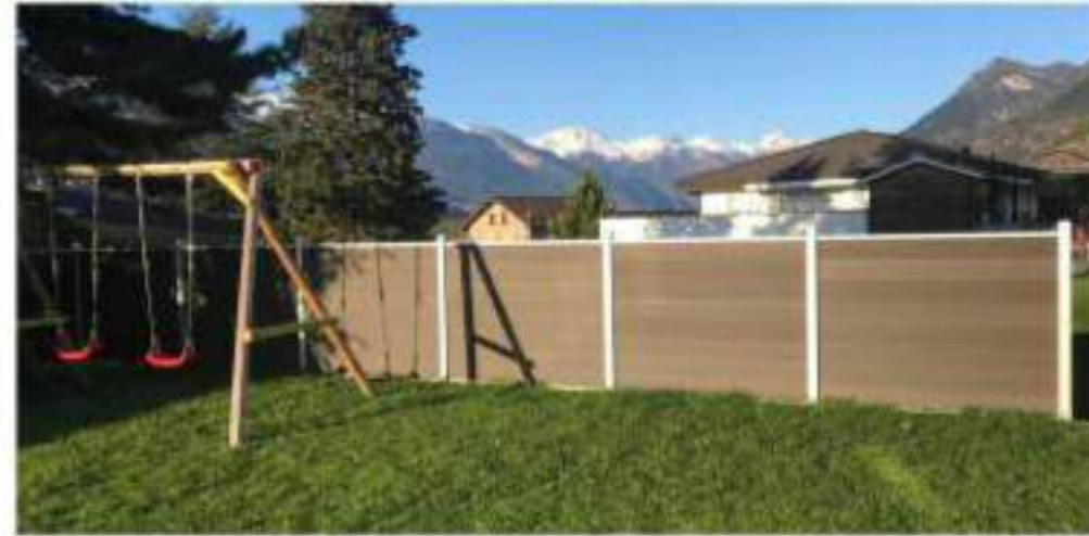
Sweden 120meters Privacy Fence Project-2019
